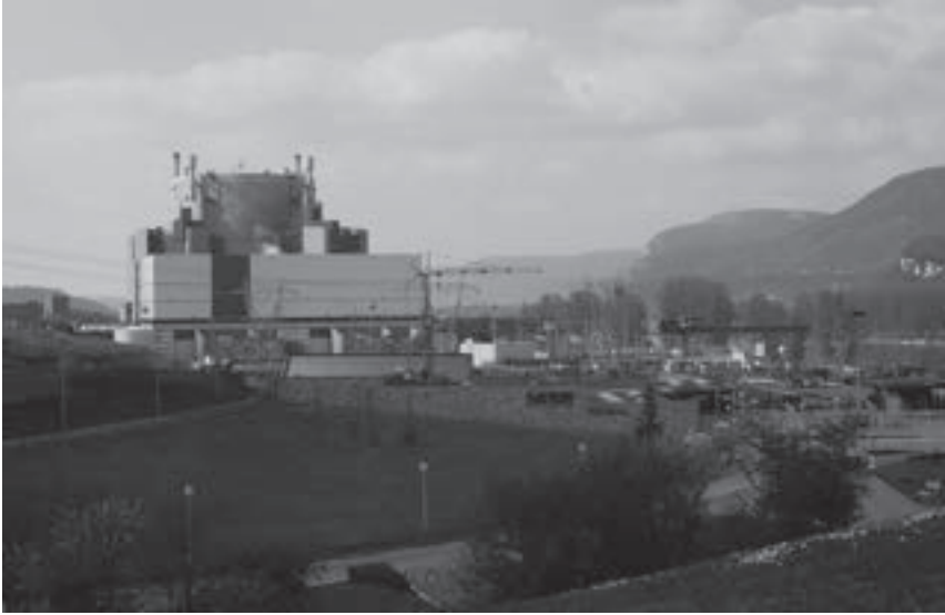
Figure 2: The almost completed Superphénix plant, 1984.
