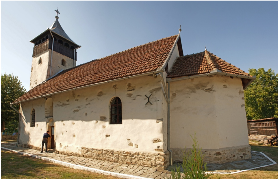
Figure 1. Crișcior church. Exterior view. Author's photo.
