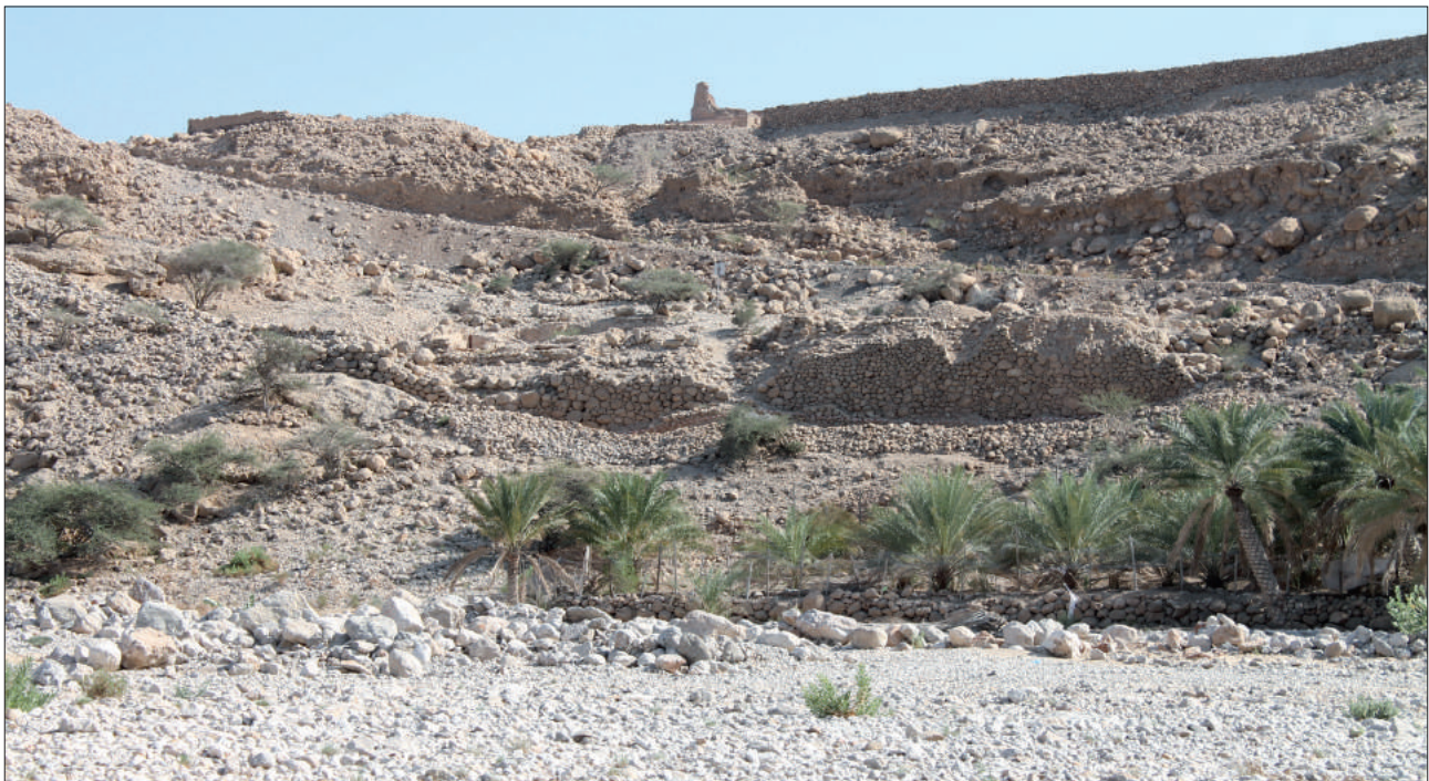
Figure 3. View from the Wādī Hilm of the northwestern gate before conservation work, the terrace, the city and wadi walls, and the modern track.
