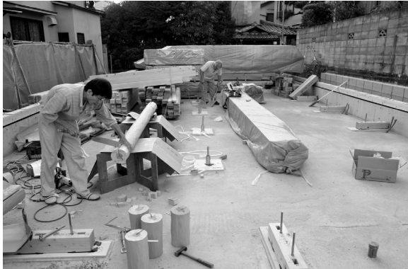
Fig. 19: Mikan, EFEO Centre Kyoto, carpenters at work, September 2013. Photograph ©Benoît Jacquet.
