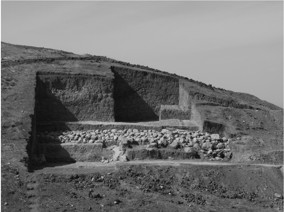
Fig. 5. Area A. The north-eastern angle of the monumental building (level 2) (C. Kepinski).
