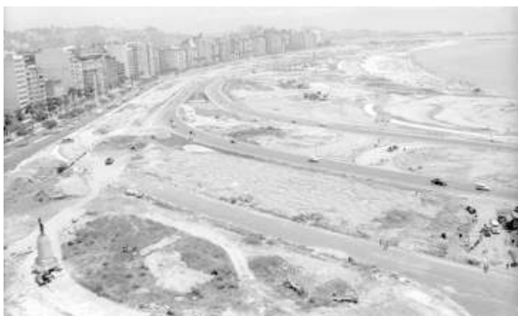
Source: O Globo archives - https://oglobo.globo.com/rio/a-construcao-do-parque-do-flamengo-17736982 .
