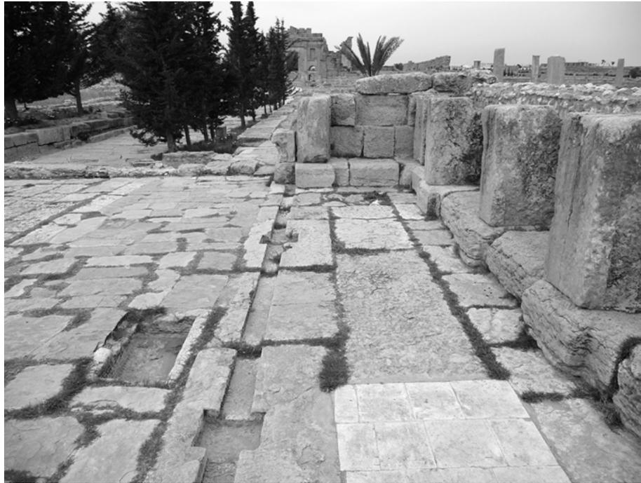
**Fig. 10:** Sbeitla, Fountain near the Basilica of Servus. In the centre, the slot where the parapet's slabs originally stood; on the left, the small tank directly below the original basin.
