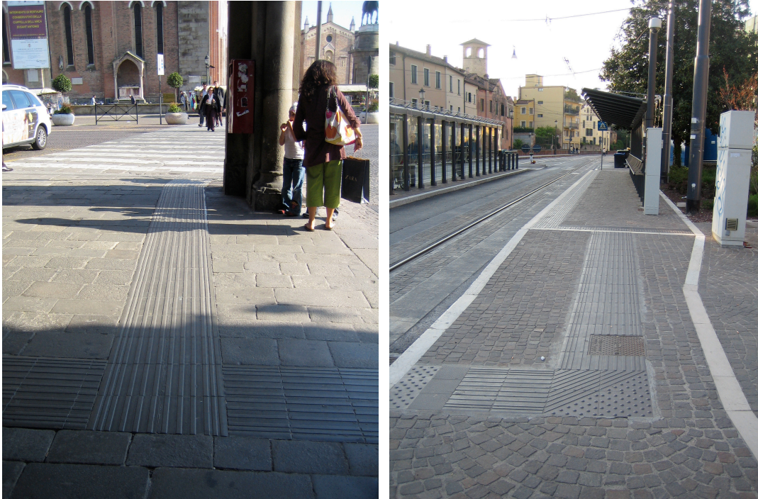
Fig. 4 & 5 - Directional strips before pedestrian crossings / Directional strips and hazard warning strips on a platform of tram (© Rachel Thomas)
