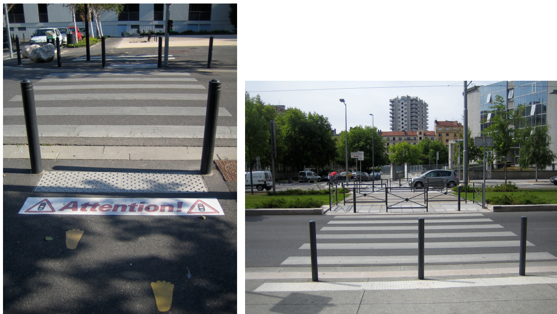
Fig. 2 & 3 - Two examples of ‘bateaux’ and hazard warning strips at pedestrian crossings (© Rachel Thomas)
