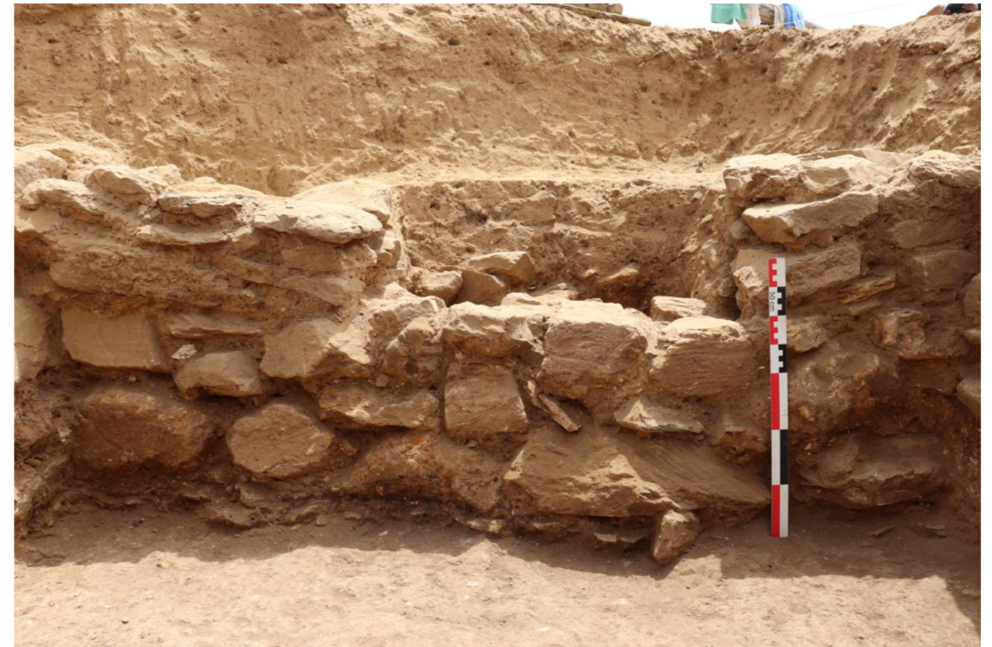
Figure 44: Gra Emni (Saz 249) - Trench 5 - Wall 249 046 with a door opening in it, between Loci 2 and 4. Looking east (G. Tavernier - MAFTOr).
