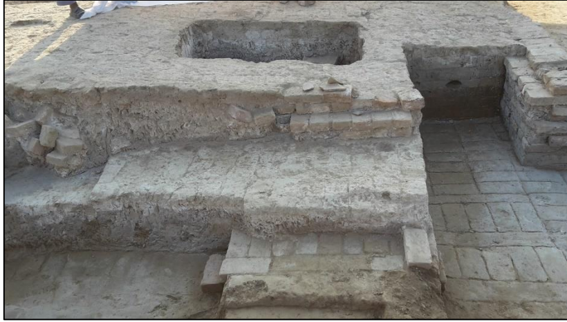
Figure 19: Trench 2 – Steps of the 'Massive Building'.
