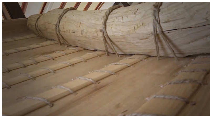
II.70 Pogled na rebro vezano za oplatu View of the frame lashed to the planking (fotografija / photo by: M. Račan)
