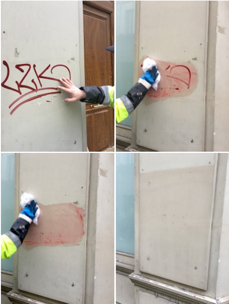
Figure 2. Making the graffiti react with chemical solvents (© J. Denis & D. Pontille)
