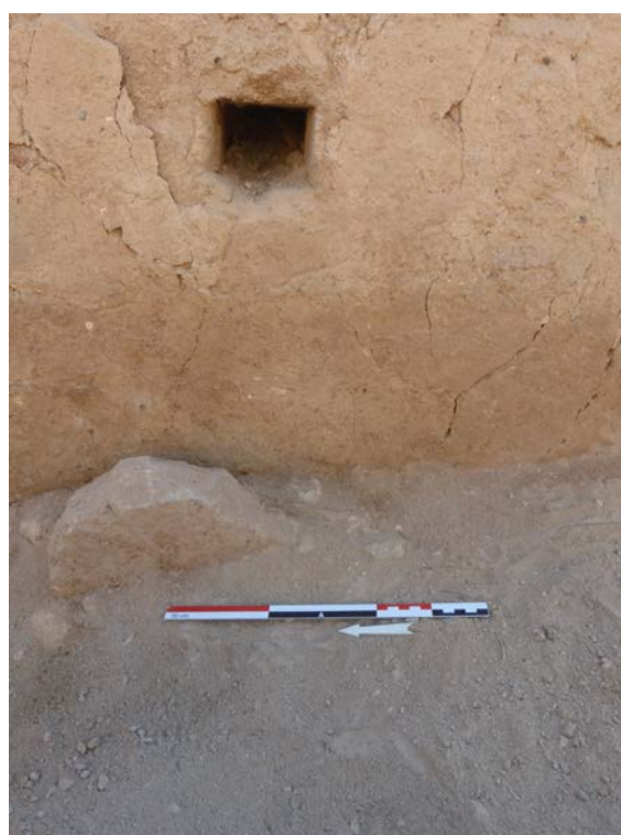
Fig. 60 - Beam hole B12-130
