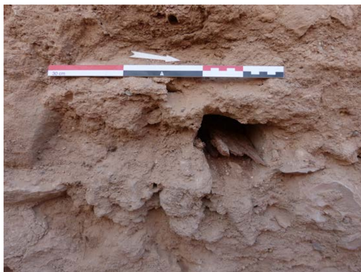
Fig. 59 - Beam hole B12-122
