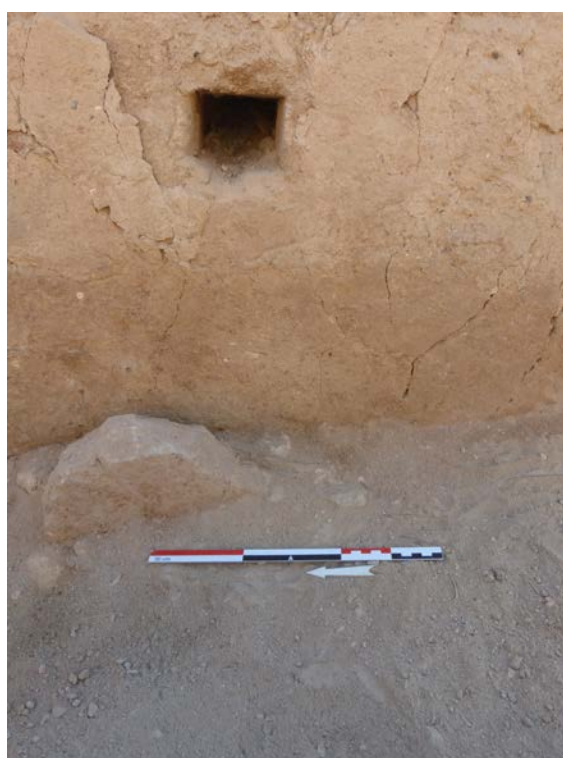
Fig. 60 - Beam hole B12-130
