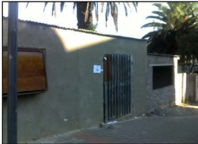
Ugly boundary wall with openings for businesses. Has the property been rezoned for business? Probably not.
