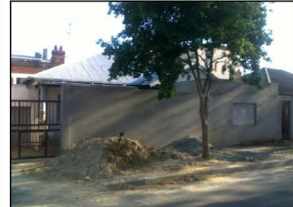
Blank wall: another example of a residential property being prepared for the installation of a spaza shop
