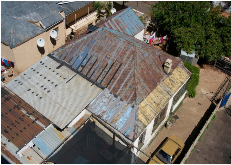
FIGURE 25.4: Thresholds: Outside room extension
