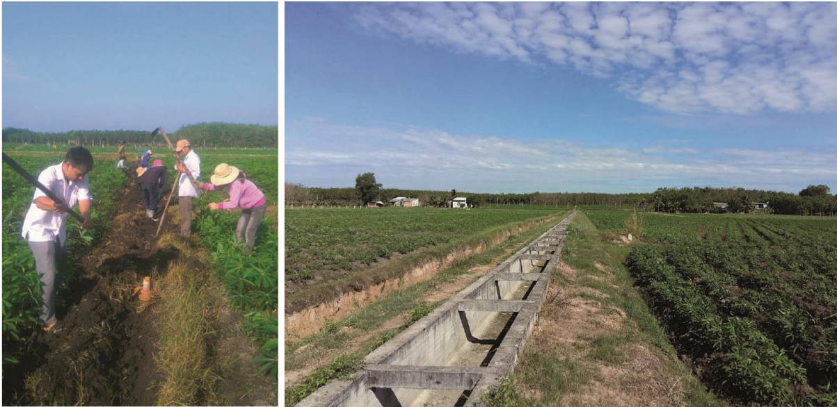
Figure 13b. On-farm canal making in the Tân-Biên perimeter: on-farm network organized by local authority at canal N2-22-1, Thanh-Tây commune.
