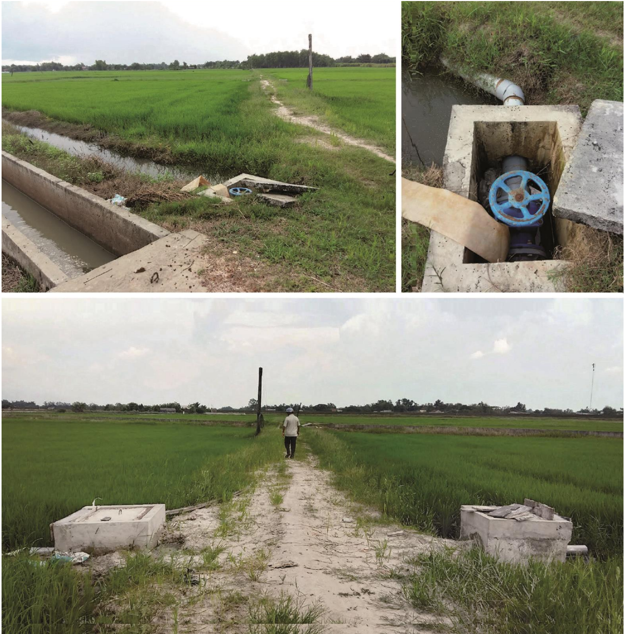
Top left: From the tertiary canal to an on-farm outlet; Top right: Outlet and on-farm canal through a pipe; Bottom: Two outlets from on-farm canals to the field. Source: EFEO, 2019.
