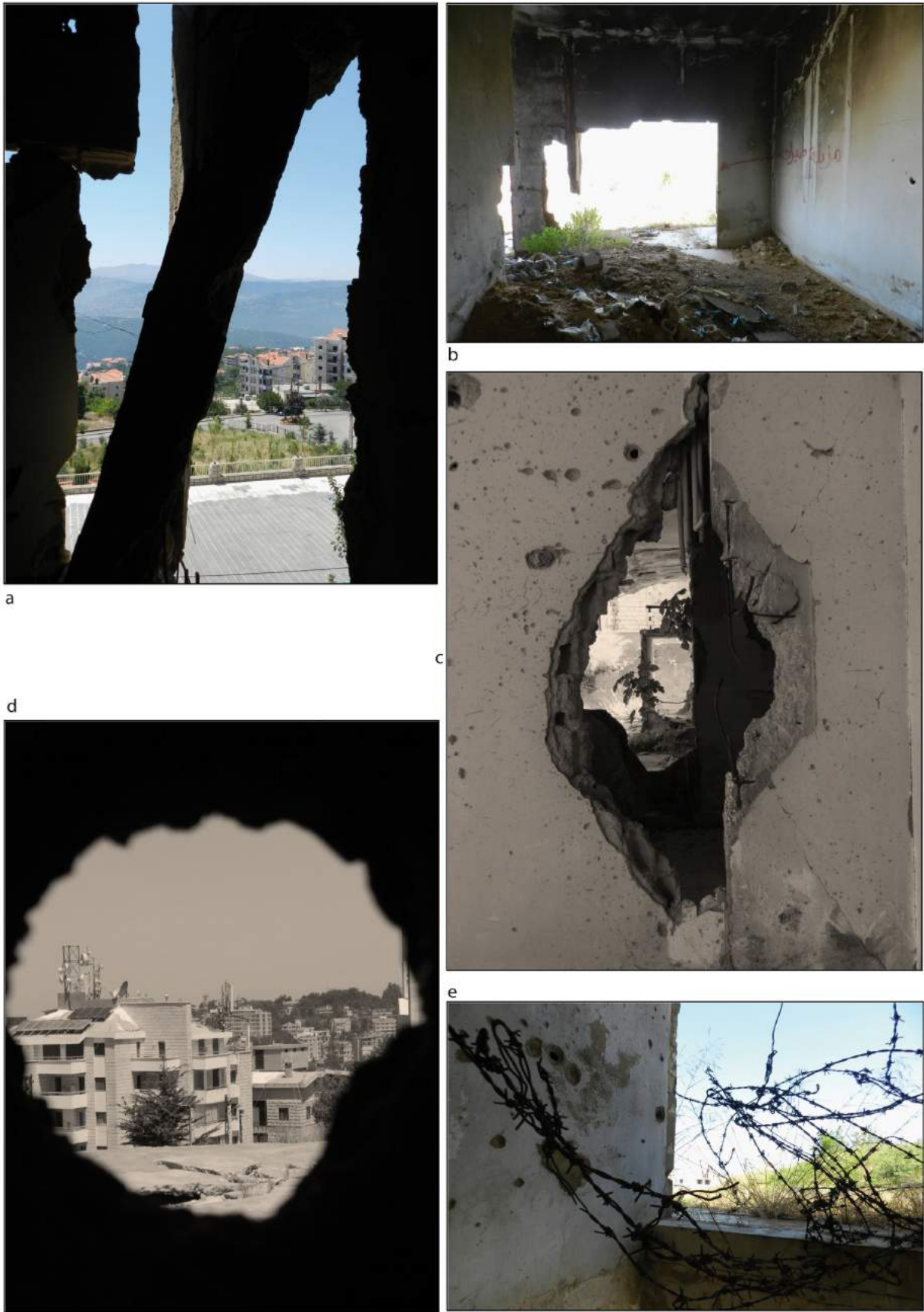
Figure 8: Qleiaat. Abandoned family homes turned into firing positions.
