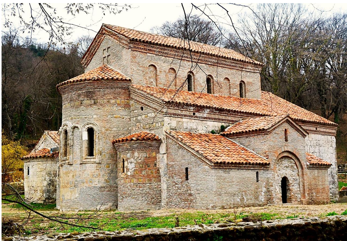
Fig. 13 (p. 407). Vazisubani, Kakheti (Georgia). Sanagire. General view from northeast. Online photograph Tengö Kekenadze
