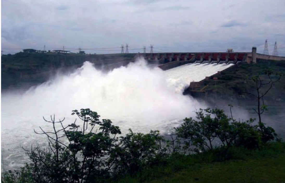
Figure 17: Spillway of Itaipu dam showing water with low sediment load, December 2010 (Francois Laurent)
